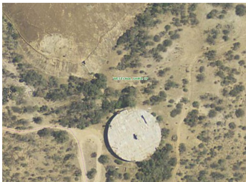
Geelakin Water Tank
