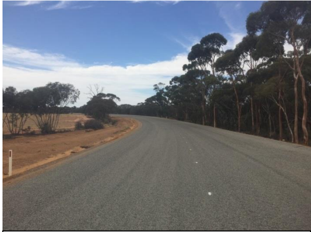
Boodarockin Rd at SLK 14.58 F – showing centre of LH curved section from SLK 14.40 to 14.94 and 10.4m seal width.
