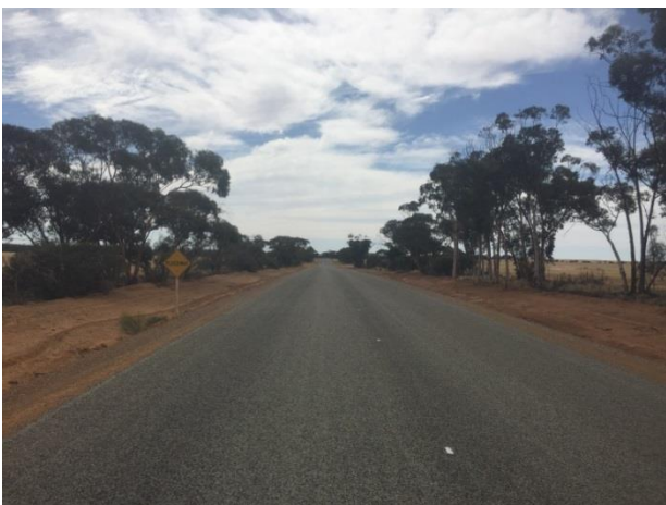
Boodarockin Rd at SLK 15.98 F – showing typical straight section from SLK 14.94 to 37.96 and 7.6m seal width.
