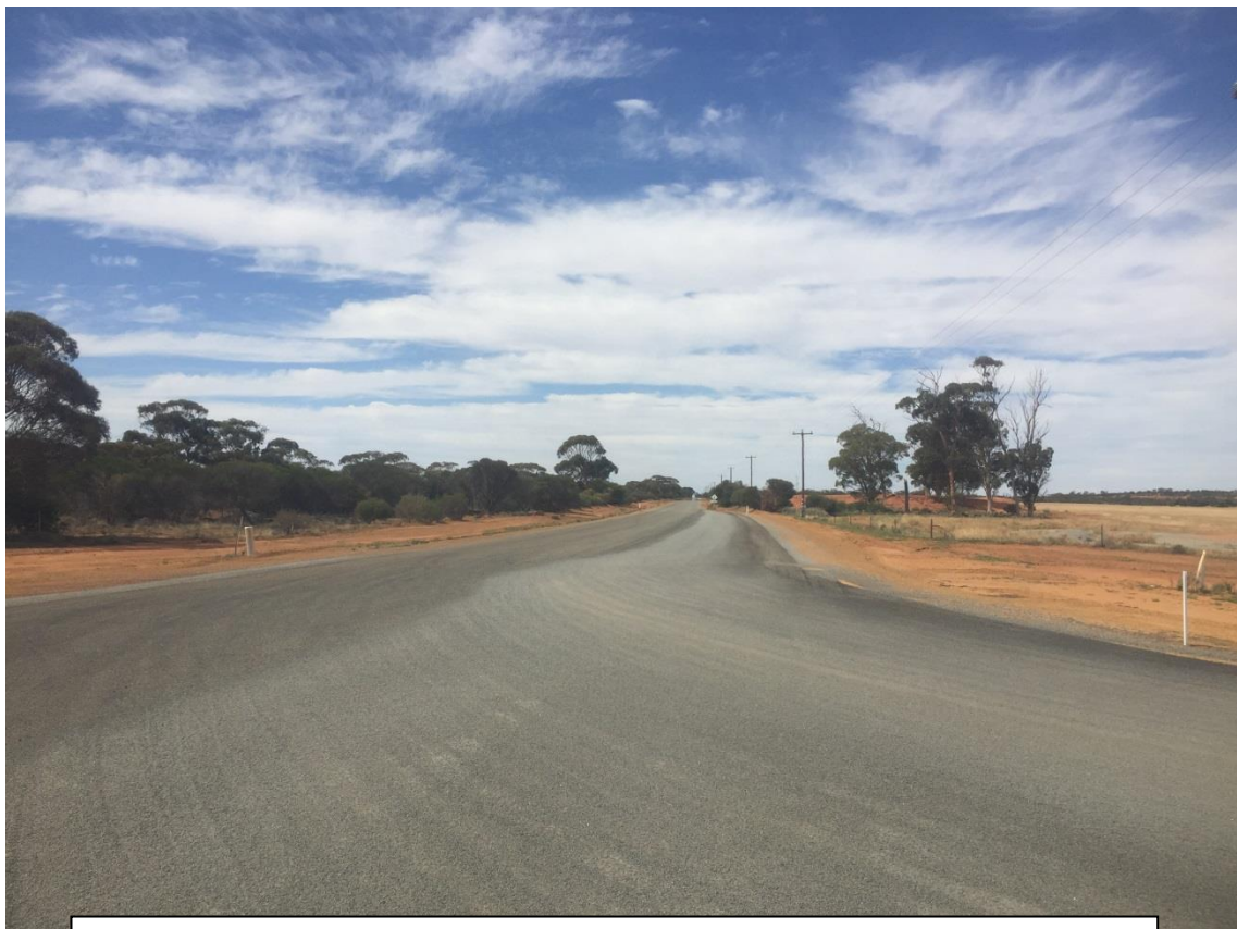
ESD Photo looking to east (RHS) at Intersection with Koorda / Bullfinch Rd at SLK 37.96 – from southern side of intersection. Photo at SLK 37.955 on Boodarockin Rd. Note the 140m long turning pocket along the southern side of the Koorda / Bullfinch Rd.
