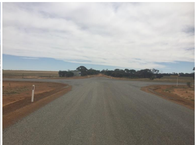
George Rd at SLK 19.22 B – showing the Cross Road intersection with Boodarockin Rd at SLK 19.18 (eastern side of the Boodarockin Rd intersection). Note : that the Giveway Sign is missing on this approach to the Boodarockin Rd Intersection and is expected to be installed by MRWA the week commencing 6 th April 2020.
