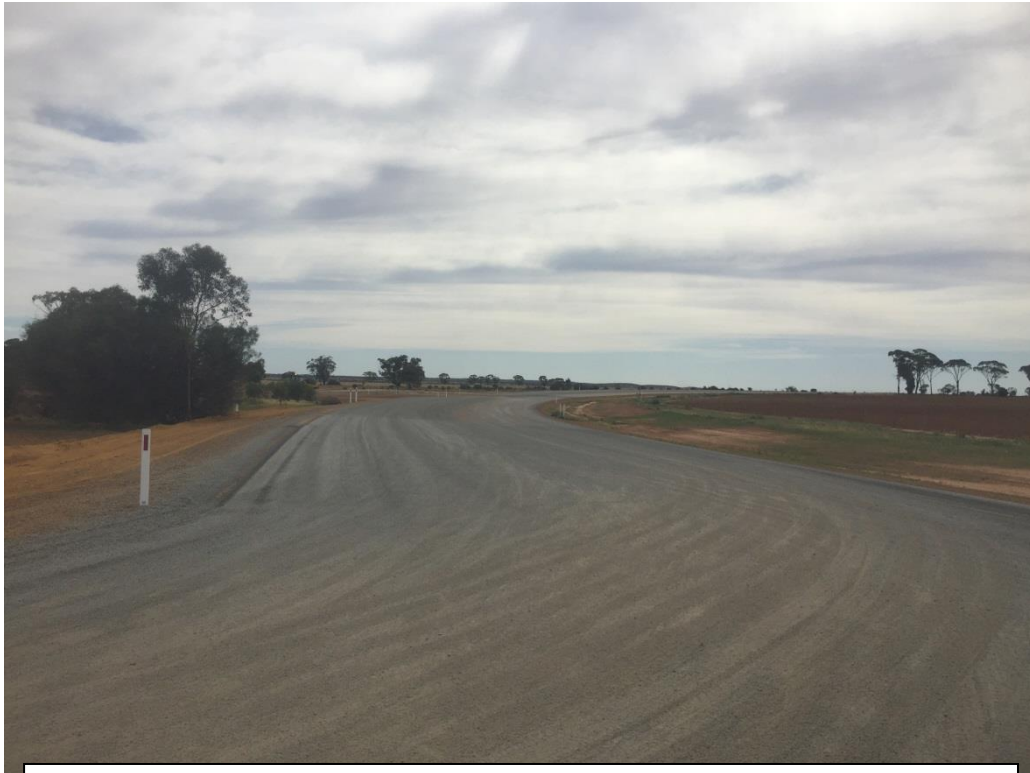
Boodarockin Rd at SLK 2.18 – showing the start of the 360m long acceleration lane from the Edna May Minesite Entrance LH T-Junction intersection at SLK 2.18.
