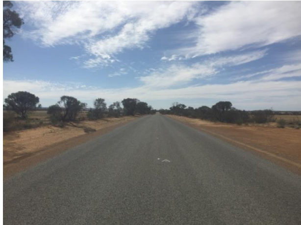
Boodarockin Rd at SLK 34.73 F – showing typical straight section from SLK 14.94 to 37.96 and 7.6m seal width.
