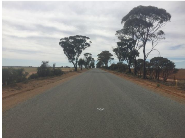
Boodarockin Rd at SLK 2.58 F – showing start of straight section from SLK 2.54 to 4.57 and 7.6m seal width.
