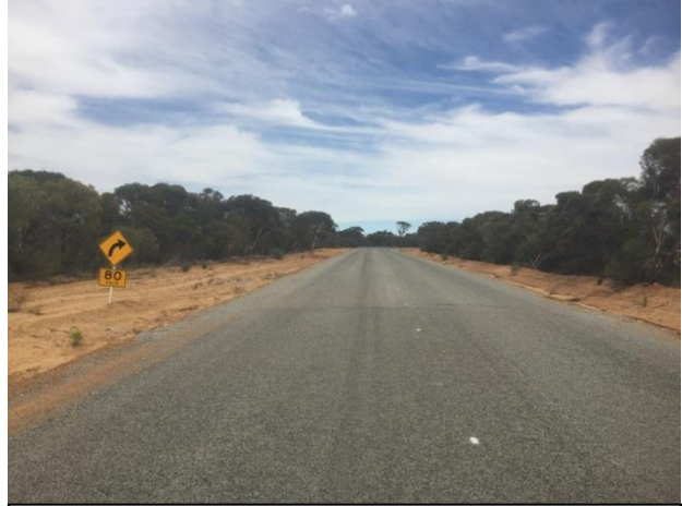
Boodarockin Rd at SLK 15.07 B – showing warning curve sign and speed advisory sign in advance of end T.P. of LH curve section from SLK 14.40 to 14.94.
