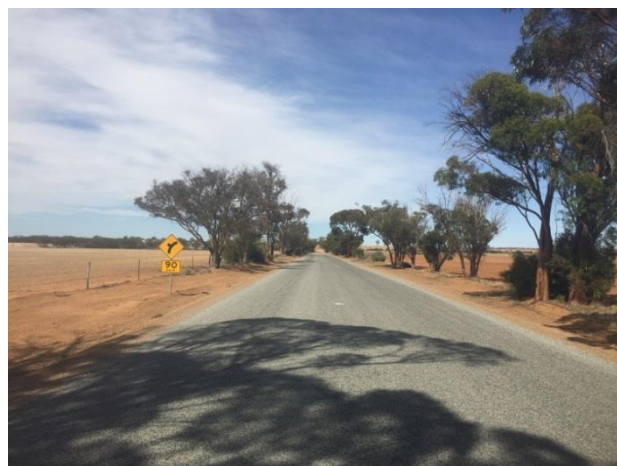
Boodarockin Rd at SLK 5.43 B – showing warning curve sign and speed advisory sign in advance of end T.P. of LH curve section from SLK 4.57 to 5.20.
