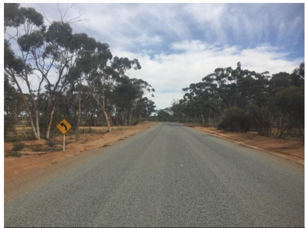
Boodarockin Rd at SLK 10.36 B – showing warning curve sign in advance of end T.P. of RH curve section from SLK 9.78 to 10.22.
