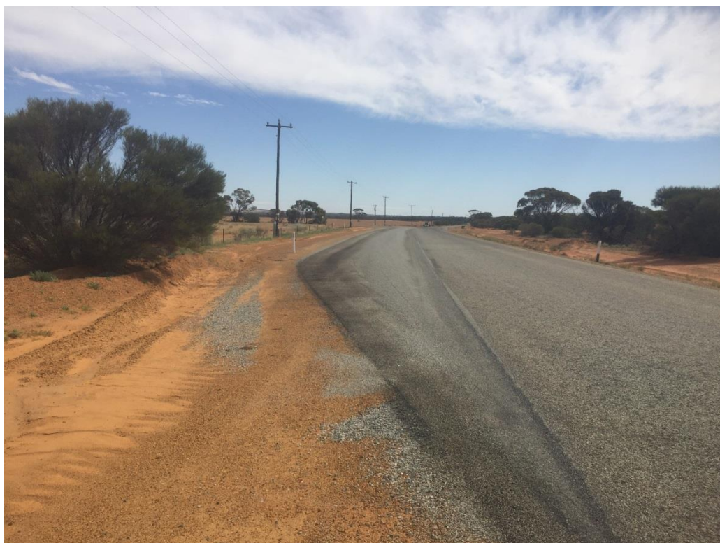
Koorda / Bullfinch Rd at SLK 28.63 B – showing the start of the Turning Pocket on the eastern approach to the Cross Road intersection with the Koorda / Bullfinch Rd at SLK 28.48. This intersection has recently been widened and upgraded to accommodate 36.5m long RAVs (7.3 / TD 4.3).
