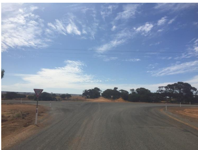
Boodarockin Rd at SLK 37.92 F – showing the Cross Road intersection with the Koorda / Bullfinch Rd at SLK 37.96. Note the Giveaway Signs installed on the Boodarockin Rd and Boodarockin North Rd approaches to the Koorda / Bullfinch Rd Intersection. This intersection has recently been widened and upgraded to accommodate 36.5m long RAVs, and includes a LH turning pocket on the eastern approach to this intersection on the Koorda / Bullfinch Rd.
