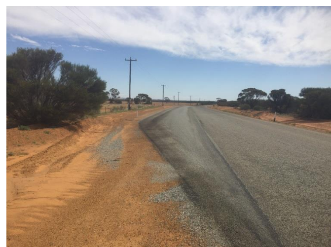
Koorda / Bullfinch Rd at SLK 28.63 B – showing the start of the Turning Pocket on the eastern approach to the Cross Road intersection with the Koorda / Bullfinch Rd at SLK 28.48. This intersection has recently been widened and upgraded to accommodate 36.5m long RAVs.
