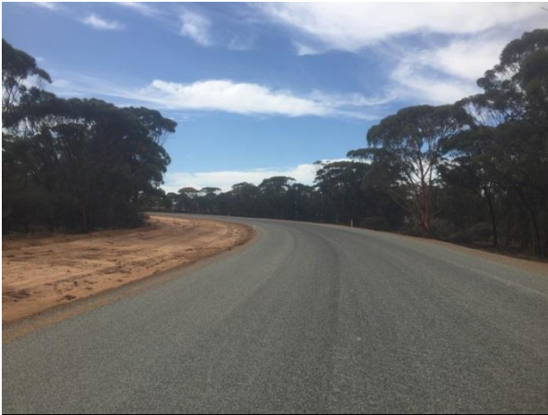
Boodarockin Rd at SLK 10.77 F – showing centre of LH curved section from SLK 10.66 to 11.32 and 10.2m seal width.
