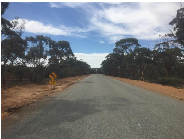
Boodarockin Rd at SLK 10.50 F – showing warning curve sign and speed advisory sign in advance of start T.P. of LH curve section from SLK 10.66 to
