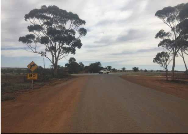
Boodarockin Rd at SLK 2.12 F – showing warning curve sign and speed advisory sign in advance of start T.P. of RH curve section from SLK 2.16 to 2.54. Note : the Edna May Gold Mine Entrance to the LHS at SLK 2.18.
