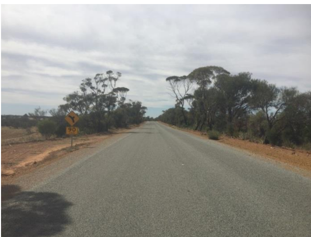
Boodarockin Rd at SLK 4.24 F – showing warning curve sign and speed advisory sign in advance of start T.P. of LH curve section from SLK 4.57 to 5.20.
