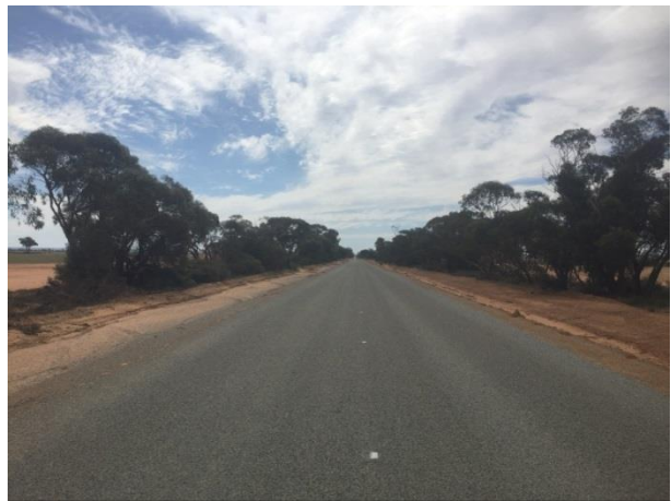
Boodarockin Rd at SLK 27.40 F – showing typical straight section from SLK 14.94 to 37.96 and 7.6m seal width.
