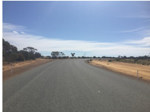
Boodarockin Rd at SLK 7.19 F – showing centre of RH curved section from SLK 7.04 to 7.52 and 10.2m seal width.
