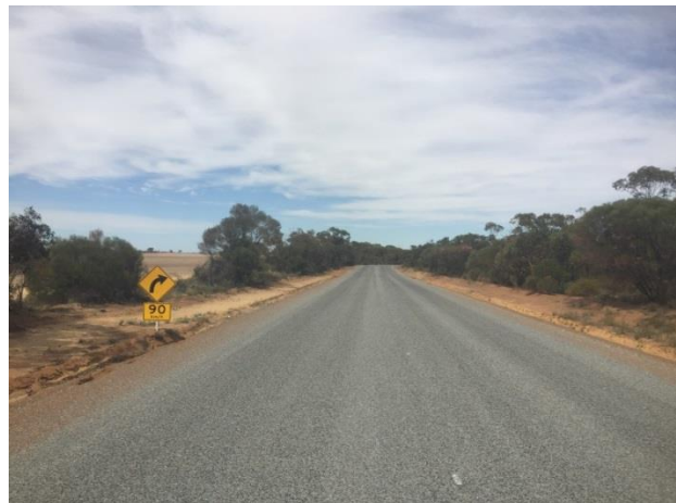
Boodarockin Rd at SLK 11.44 B – showing warning curve sign and speed advisory sign in advance of end T.P. of LH curve section from SLK 10.66 to 11.32.
