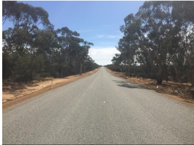
Boodarockin Rd at SLK 12.52 F – showing typical straight section from SLK 11.32 to 13.18 and 7.6m seal width.
