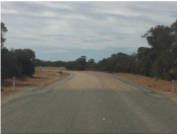
Boodarockin Rd at SLK 4.56 F – showing start of LH curved section from SLK 4.57 to 5.20 and 8.6m seal width.
