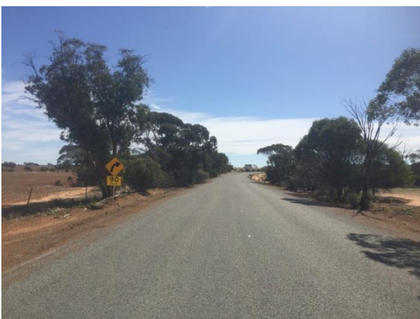
Boodarockin Rd at SLK 6.98 F – showing warning curve sign and speed advisory sign in advance of start T.P. of RH curve section from SLK 7.04 to 7.52.
