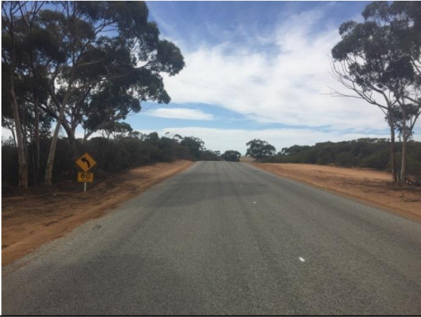
Boodarockin Rd at SLK 14.23 F – showing warning curve sign and speed advisory sign in advance of start T.P. of LH curve section from SLK 14.40 to
