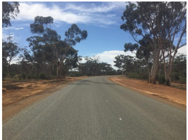
Boodarockin Rd at SLK 10.06 F – showing centre of RH curved section from SLK 9.78 to 10.22 and 10.2m seal width.
