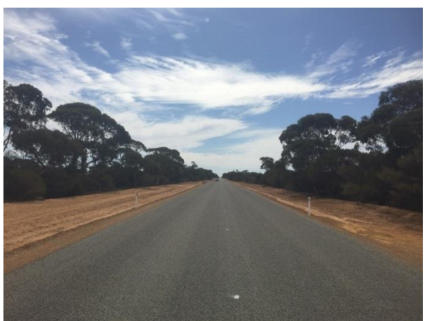
Boodarockin Rd at SLK 20.37 F – showing typical straight section from SLK 14.94 to 37.96 and 7.6m seal width.
