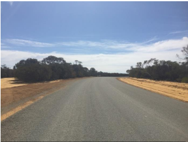
Boodarockin Rd at SLK 13.37 F – showing centre of RH curved section from SLK 13.18 to 13.88 and 10.6m seal width.
