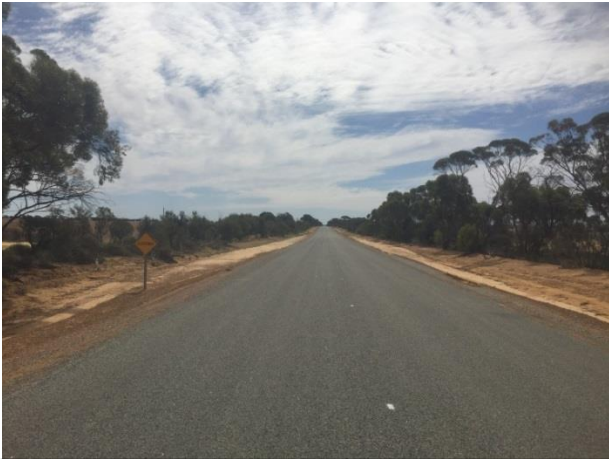
Boodarockin Rd at SLK 24.18 F – showing typical straight section from SLK 14.94 to 37.96 and 7.6m seal width.
