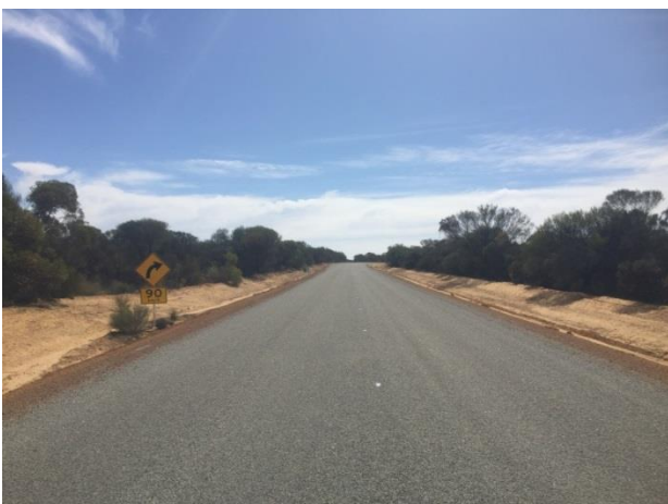
Boodarockin Rd at SLK 13.04 F – showing warning curve sign and speed advisory sign in advance of start T.P. of RH curve section from SLK 13.18 to
