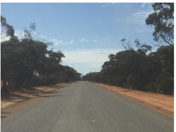
Boodarockin Rd at SLK 37.34 F – showing typical straight section from SLK 14.94 to 37.96 and 7.6m seal width.
