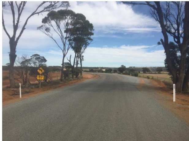
Boodarockin Rd at SLK 2.58 B – showing warning curve sign and speed advisory sign in advance of end T.P. of RH curve section from SLK 2.16 to 2.54.
