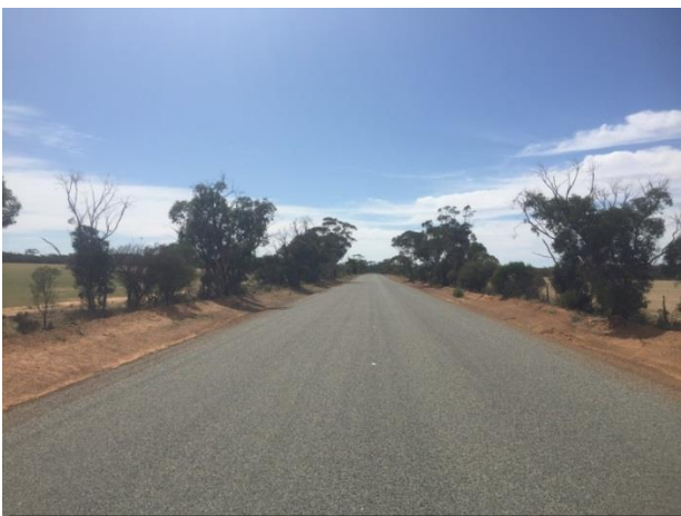
Boodarockin Rd at SLK 9.04 F – showing typical straight section from SLK 7.52 to 9.78 and 7.6m seal
