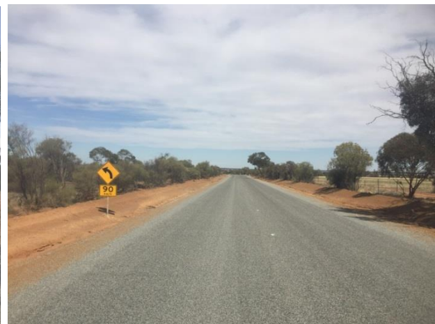
Boodarockin Rd at SLK 7.70 B – showing warning curve sign and speed advisory sign in advance of end T.P. of RH curve section from SLK 7.04 to 7.52.
