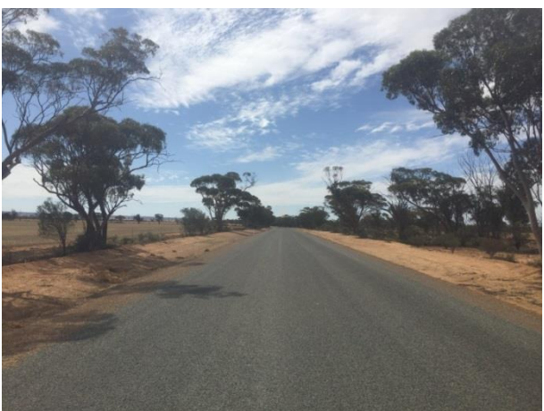
Boodarockin Rd at SLK 36.23 F – showing typical straight section from SLK 14.94 to 37.96 and 7.6m seal width.
