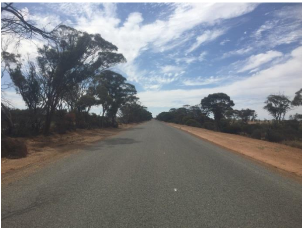
Boodarockin Rd at SLK 31.64 F – showing typical straight section from SLK 14.94 to 37.96 and 7.6m seal width.
