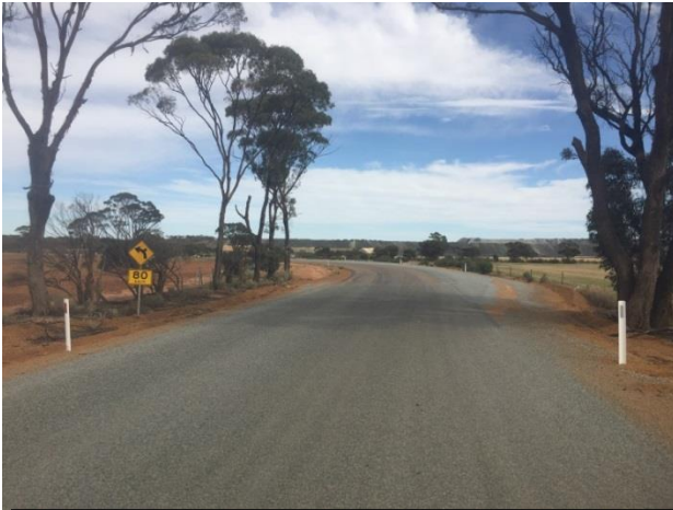
Boodarockin Rd at SLK 2.58 B – showing end of acceleration lane and 12.6m wide seal width section through RH curve from SLK 2.18 to 2.54.
