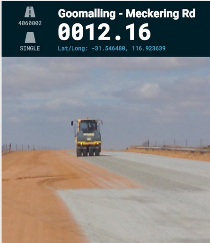
[Photo: Goomalling - Meckering Rd Project 2021/22]
