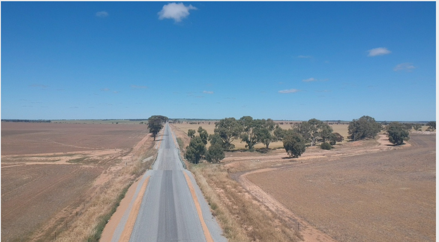
[Photo: Merredin - Narembreen Rd Project 2020/21]
