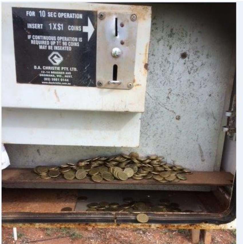
Figure 9: Inside a coin operated standpipe controller
