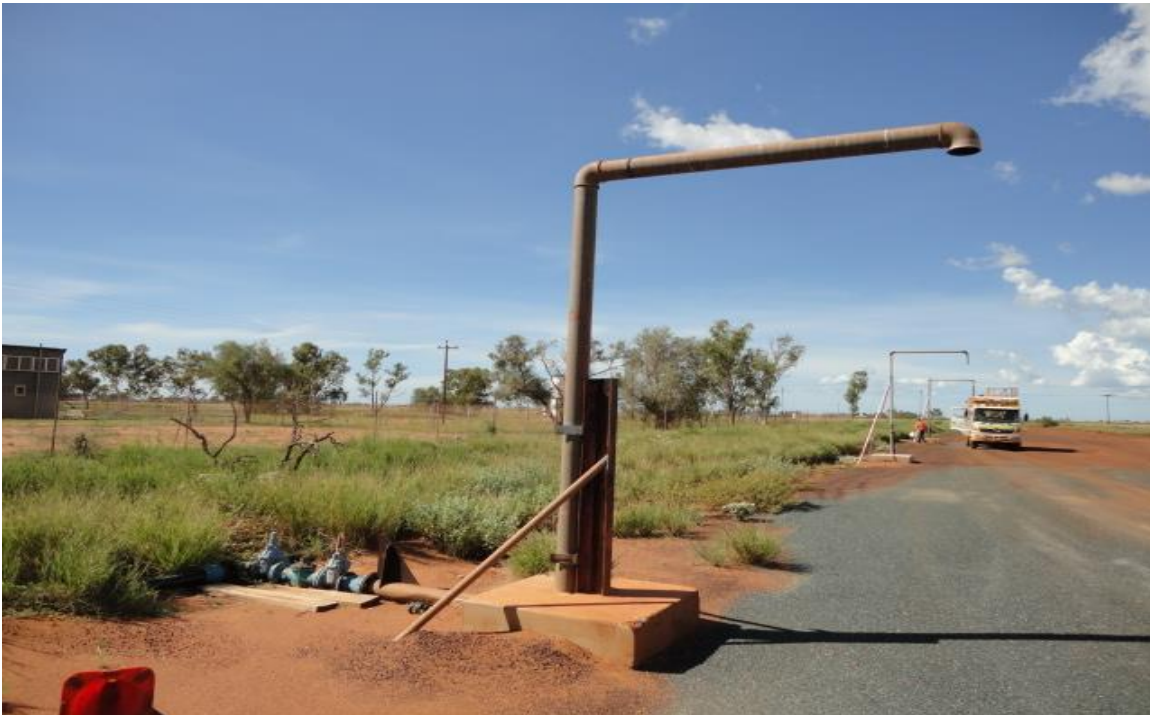
Figure 4: A row of standpipes in the North West Region
