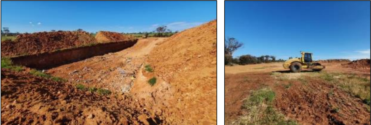
Figure 3.8 - Current landfill trench and rubbish compactor
