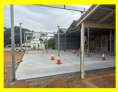
The Warm Water Pool concrete structure has been poured and will be left to cure for a month or so. Building structural works will commence soon in between the building works being carried out at the new Museum.
