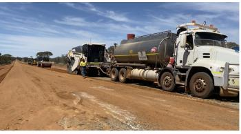
A 4km section of South Walgoolan Road has Heather's role is to facilitate a range of financial been treated with a polymer product that assists in the increased binding of gravel surfaces that helps to reduce corrugations and dust in the longer term.
