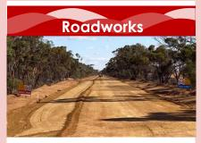
The construction crew have been making huge headway into the Boodarockin Road Sealing Project. A total of 28km of the road will have been reconstructed and 2 coat bitumen sealed. The gravel carting road trains have also made huge headway on the northern portion of the project on the final 7km of gravel heaps which will be levelled over the coming week.
